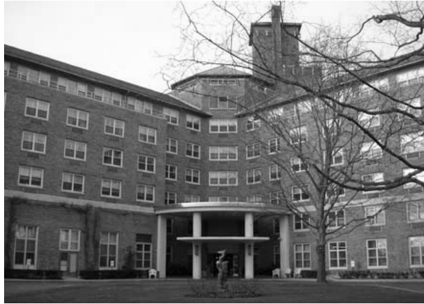
Front View of AOH
